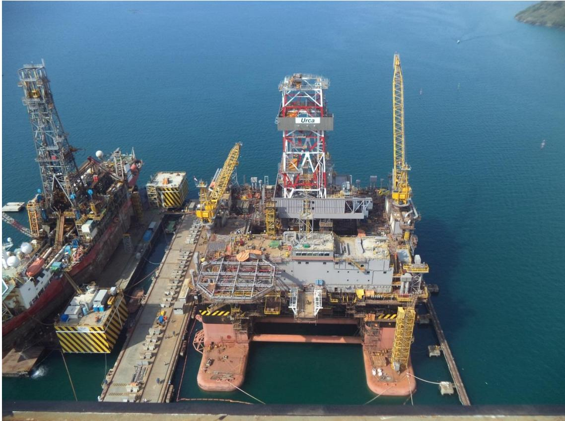
**The Urca rig, which is under construction at the Brasfels shipyard, is 82% complete. It weighs 26,500 tons and will have 55% local content.**
